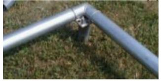
3. Then join the joiner pipe to the other end of the first pipe, and the second pipe onto the joiner pipe. Proceed around the square to complete the assembly.
